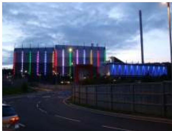
Figure 24: Plymouth Energy Recovery Facility
