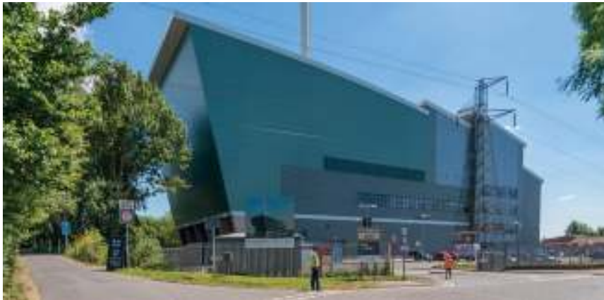
Figure 23: Exeter Energy Recovery Facility
